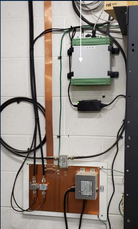
Leica GR-50 Receiver
